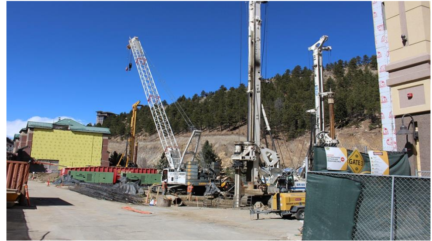
Hotel Tower/Casino Expansion: Current Progress
