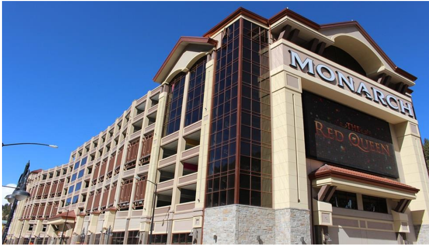
New Parking Structure
